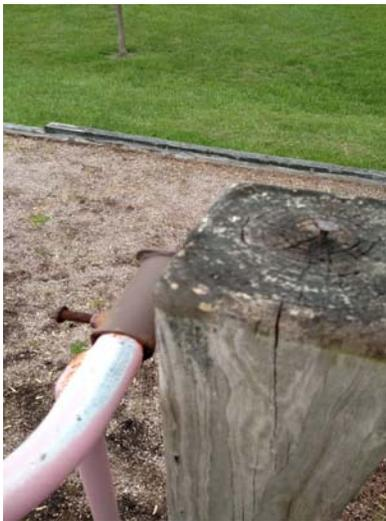
Exposed nail on handrail post
